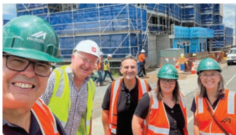
↑ The Salvos team inspecting progress during the building of the project.
